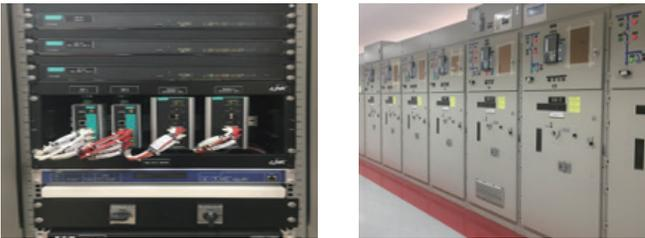
The upgrade consisted of a Moxa IEC 61850 PRP/HSR redundant network, which enables substations to operate automatically and achieve real-time communication. This process makes it possible, for example, for one substation to take over if another one is disabled due to severe weather or an automobile collision. The resulting network dependability ensures reliable communication with zero packet loss and zero-time recovery.
